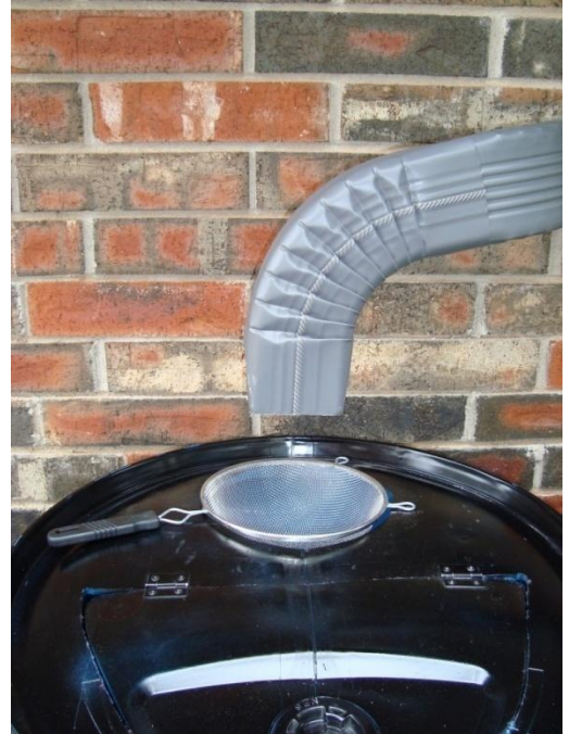
Hole in barrel for water inlet. Colander strains leaves. Hinged half-moon access panel is cut in top of barrel.
