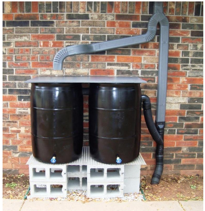
Complete system with plywood guard on top of barrels to protect from leaves. Flex hose from barrel outlet connects to plastic Y-adapter.
