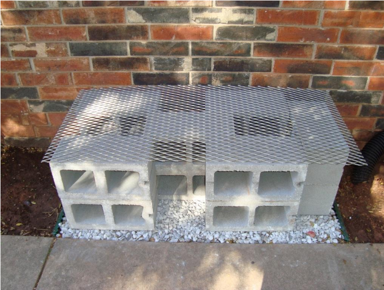
Foundation of sand, gravel, cinder blocks, and a sheet of expanded metal.
