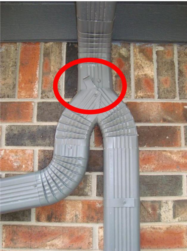
Y-shaped diverter section in 3" x 4" downspout. Lever diverts water either toward barrels or underground drain.
